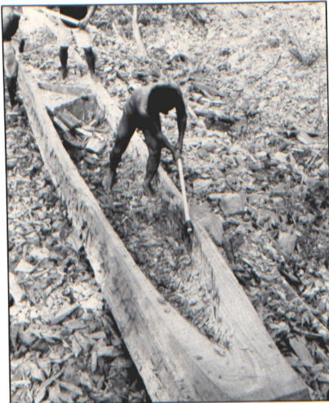
Emberá carpenters are masters with the axe, removing a maximum amount of wood with a minimum amount of work.
